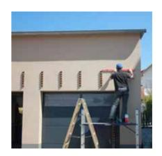
Install battens vertically and levelled in horizontal direction.
